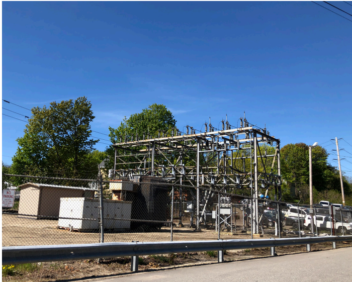
Beginning in August 2020, CMP will be upgrading its aging low-voltage substation with new equipment and mitigate the property to address flood surge issues.
